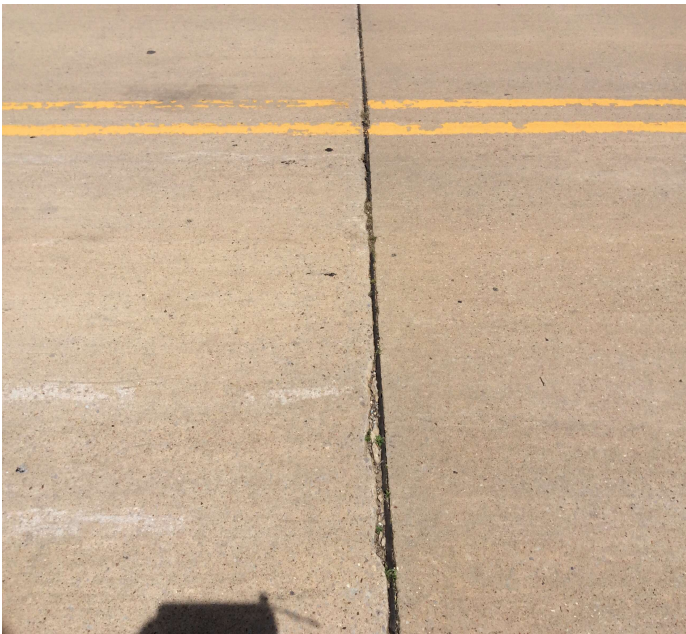
PHOTO 1 Description Deck joint sealant
