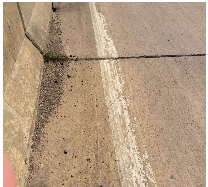
PHOTO 2 Description Diagonal cracking over Bent 3.
